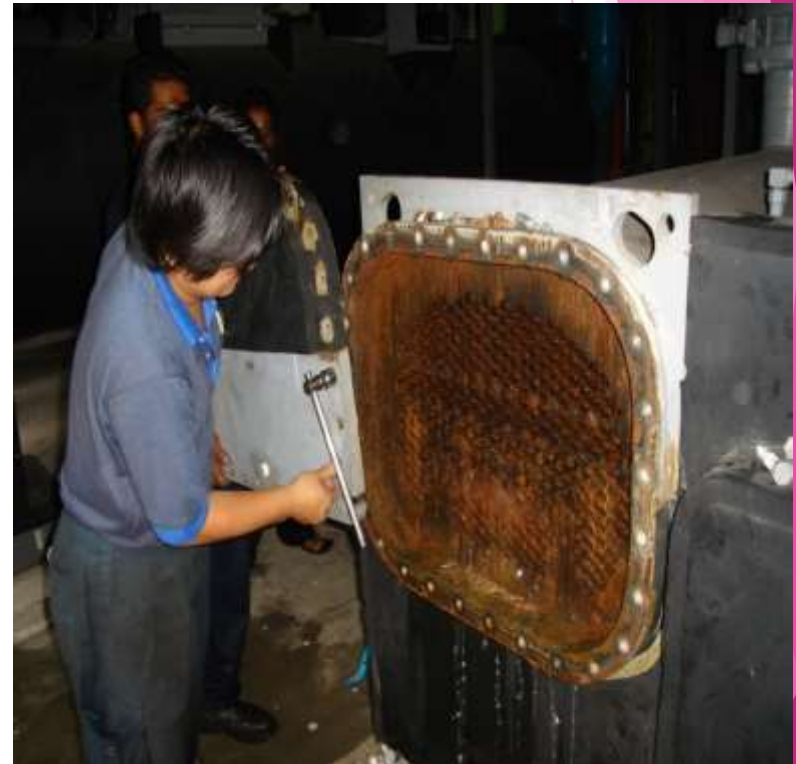
PENCUCIAN CONDENSER TUBE
