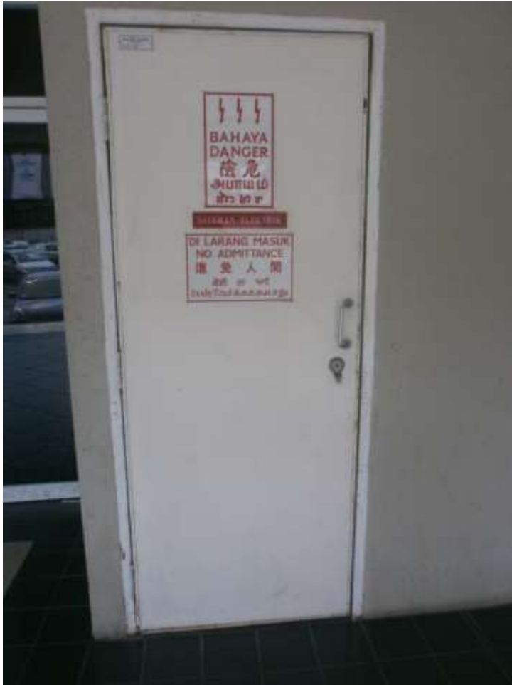
LEVEL 1,2,3 & 4 ELECTRICAL RISER ROOM
